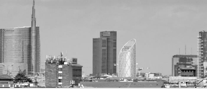
Torre Unipol, Milano
